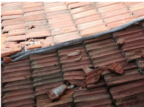
Damage of Convent Roof Tiles
