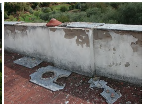
Damage to Terrazzo wall at the convent
